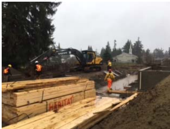
Carpentry Foundation Ace-It students at Habitat for Humanity building site in Campbell River
