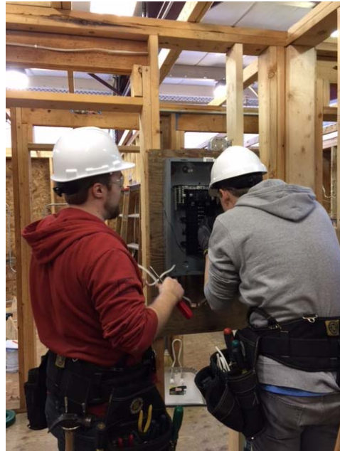
Electrical Foundation Students working on mock-up in CR
