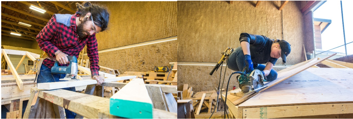
Carpentry Foundation students are working in the CV Carpentry Shop on the Hip Rafters for a Hip Roof.
